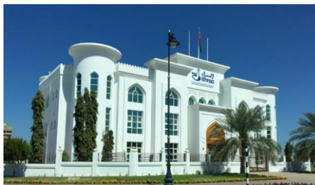
The Public Authority for Investment Promotion and Export Development building in Muscat.
